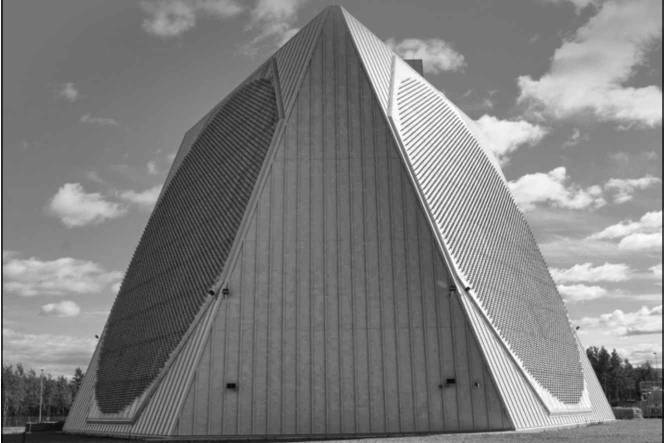
The 11-story tall Solid-State Phased Array Radar System (post Cold War missile warning system), Clear Air Force Station, Alaska.
