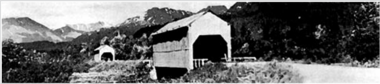
Twin covered bridges were built north of Seward in 1928. Photo courtesy Alaska State Library-Historical Collections.
