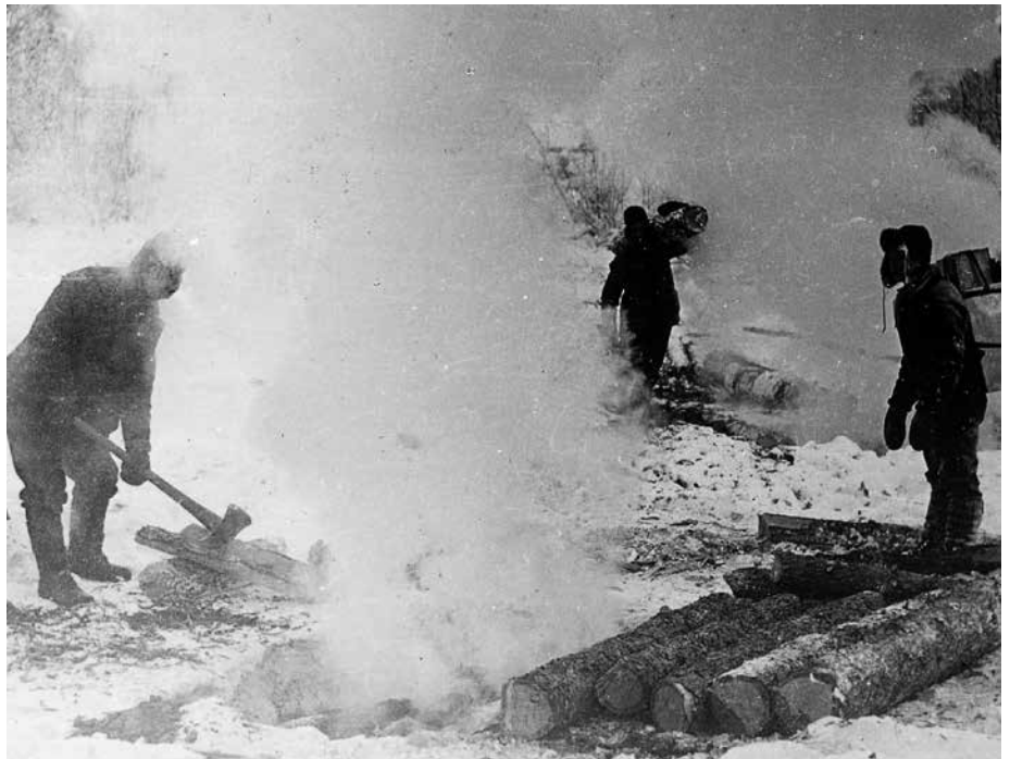
Gold miners splitting wood to feed the fire in their prospecting shaft, ca. 1898. From glass lantern slide, courtesy of Chris Allan.
