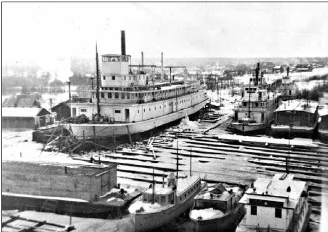
SS Nenana being built, 1932. Photo courtesy Pioneers of Alaska Museum of Fairbanks, Bill Berry Collection.
