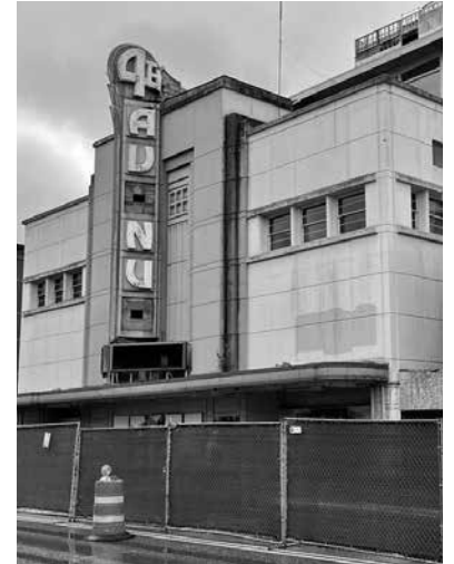
Fourth Avenue Theatre with demolition underway. Photo by Darrel Hess.
