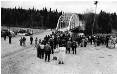
Bridge over the Kenai River, 1952. Photo by Les Anderson via Wikipedia; public domain.
