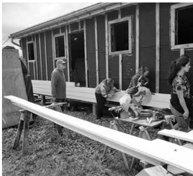
Volunteers put siding on the Japonski boathouse. Photo courtesy Sitka Maritime Heritage Society.
