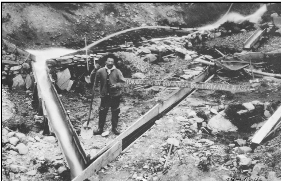
A placer miner on Bonanza Bar of the Fortymile River uses a hydraulic cannon to push gold-rich gravel into sluice boxes, ca. 1915. University of Alaska Fairbanks, George King Collection (19898-131-46).
