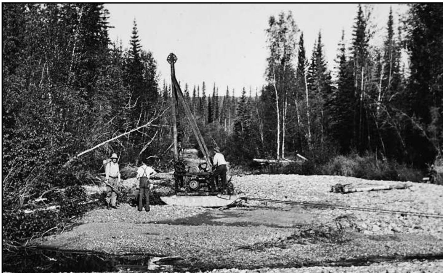
Workers at Coal Creek use a mobile "Airplane" drill to test gravel for gold values. The drill was designed by C. Kirk Hillman of Seattle to be light enough that the disassembled unit could be dropped from an airplane into remote locations. (SP)
