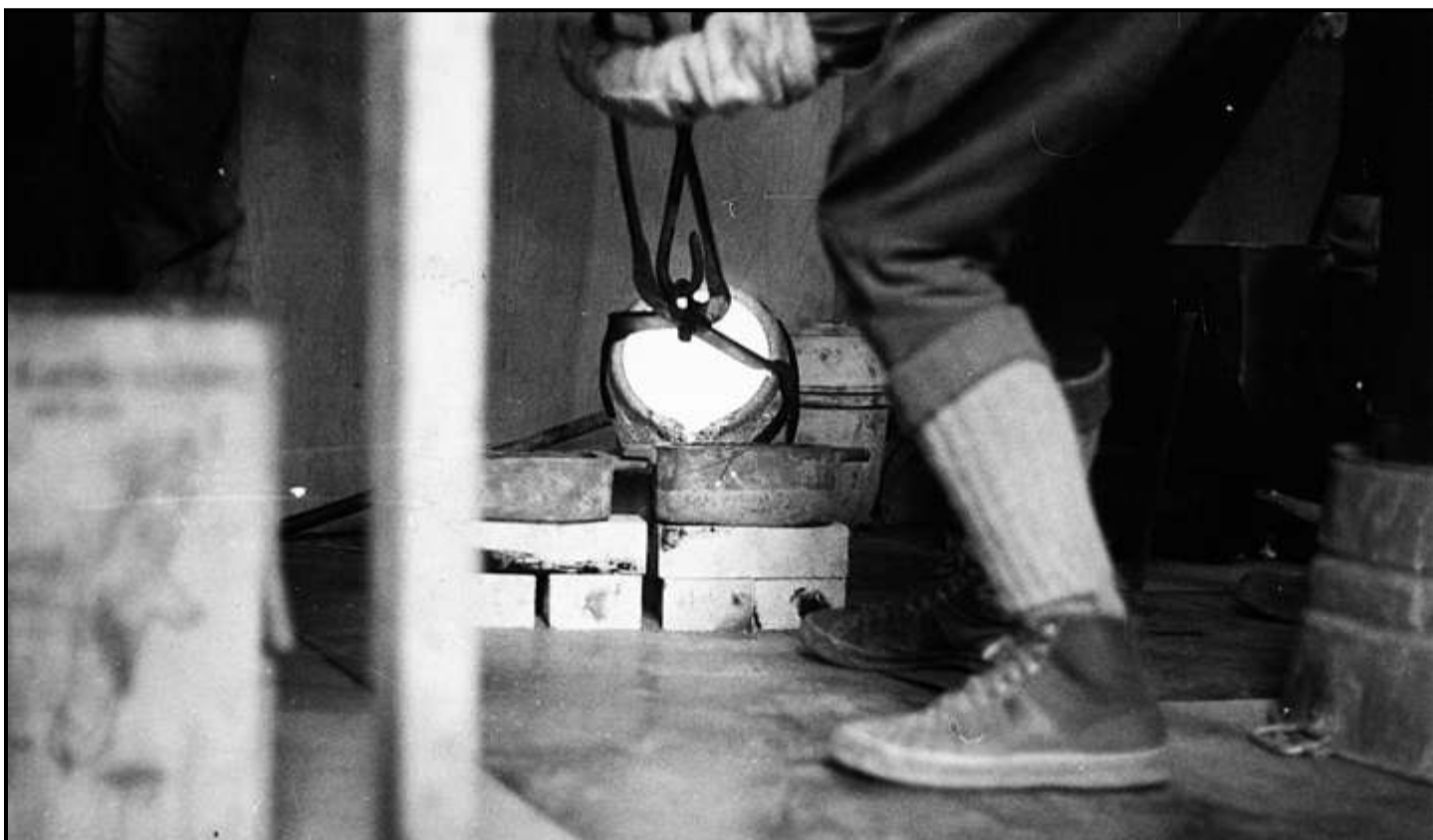
The “sponge” is heated a second time in a crucible until it is molten. Once the gold is poured into a mold, impurities called “slag” can be chipped away and the gold bar is sent by U.S. Postal Service to a bank in Seattle, Washington. (SP)
