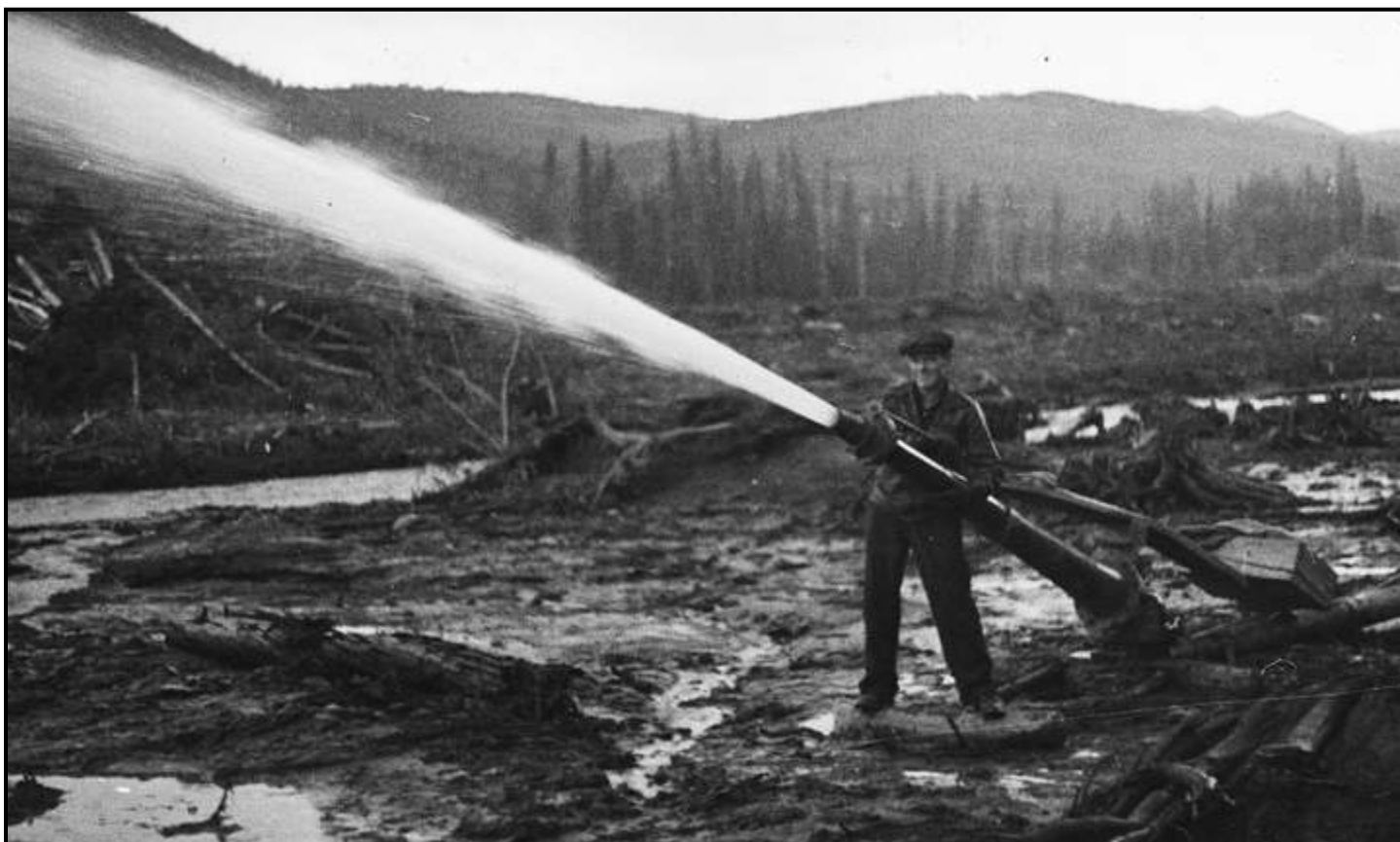
A dredge employee uses a hydraulic cannon, or giant, to strip away the ground's organic layer and accelerate thawing in advance of the dredge. At the rear of the nozzle are counter-weights to help the worker handle the power of the cannon. (AH)
