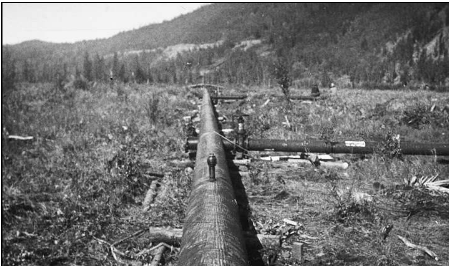
An elaborate system of hydraulic piping was used to transport water for giants and thawing points. The points, made of rubber hose and steel pipe with a chisel bit, were driven into frozen ground, inches at a time, to melt many acres of permafrost. (SP)
