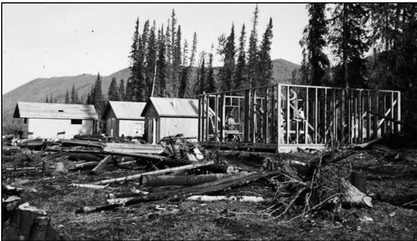
These bunkhouses were built on log skids equipped with steel cables that made it possible for tractors to relocate the entire camp to be closer to the gold dredge as it moved up and down the Coal Creek drainage. (SP)
