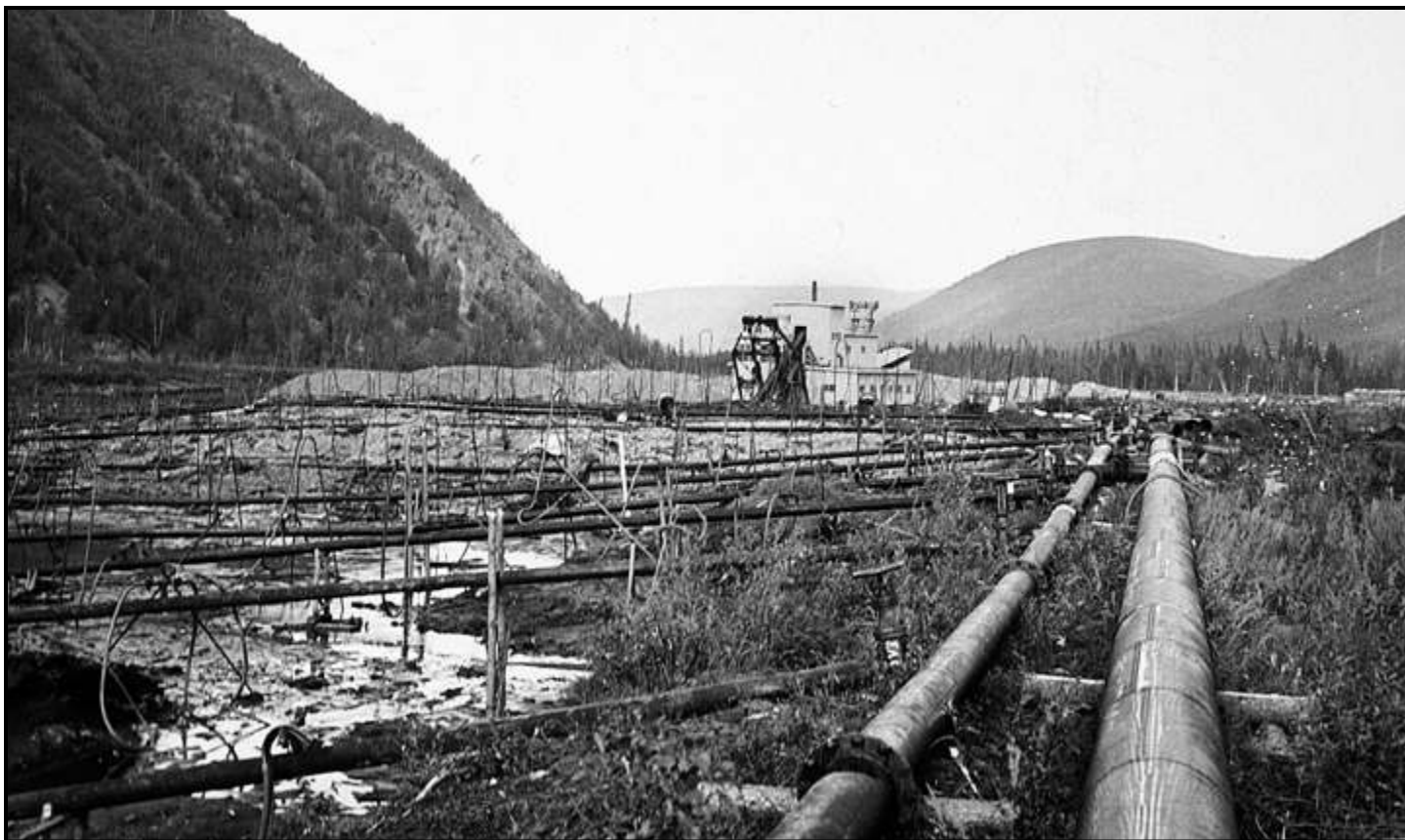
A field of thawing points used to inject air-temperature water into the ground to melt permafrost. This work needed to be done the year before the dredge arrived to ensure that thawing had reached at least twenty-five feet of depth. (SP)
