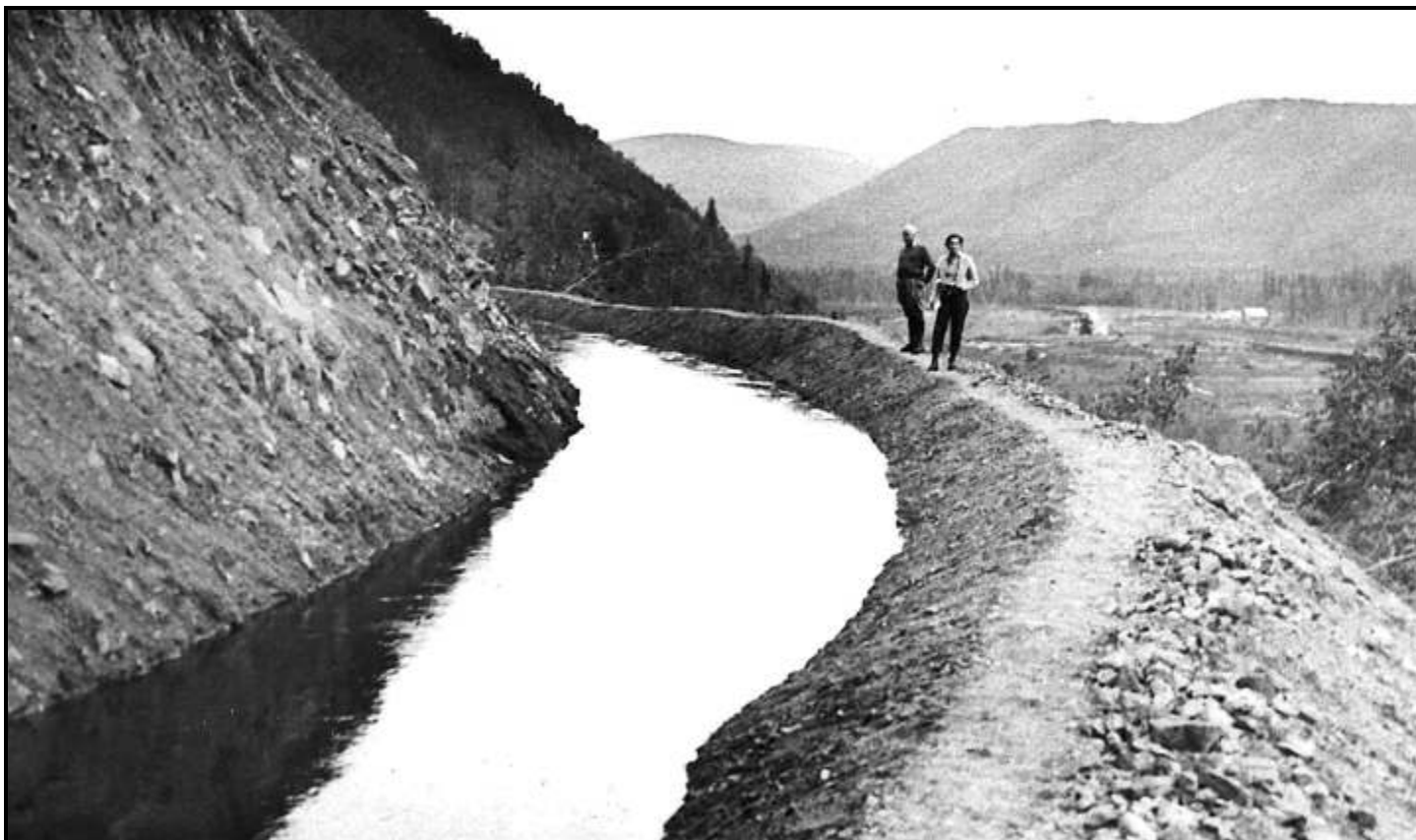
Ernest Patty and his wife Kathryn stand along the two-mile ditch above Coal Creek. The ditch provided water under pressure for stripping and thawing in advance of the gold dredge. (EP)
