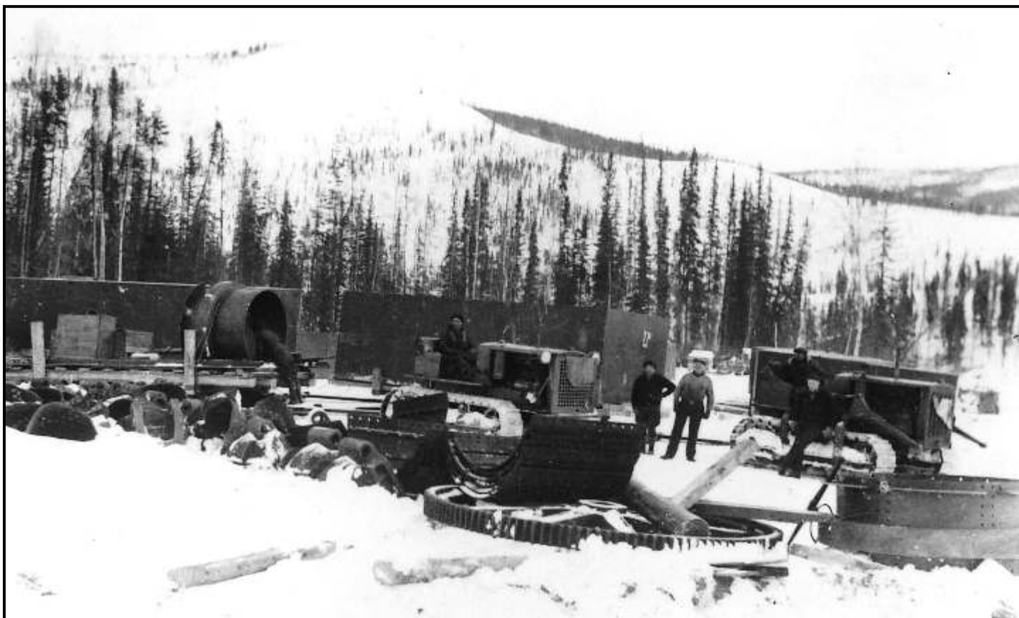
Dredge buckets and sections of the trommel (the dredge's main gravel-washing mechanism) lie in the snow, waiting to be transported to the construction site. In all, the parts, tools, and other equipment weighed about 400 tons. (EP)
