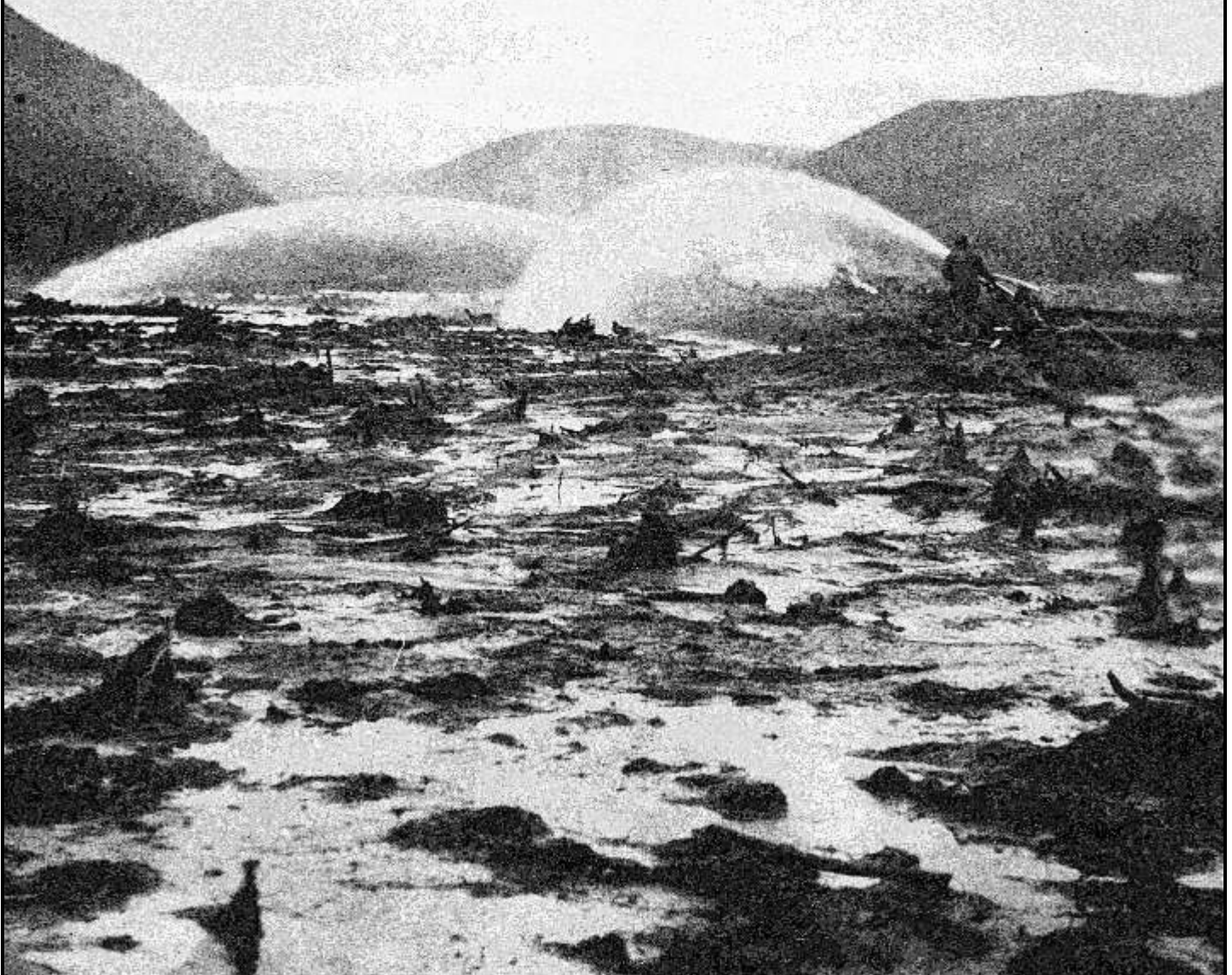
A battery of hydraulic cannons, called giants, strip away the organic material (called muck) to begin thawing the permafrost below. This ground preparation was essential because the dredge's buckets would be damaged by frozen gravel. (EH)
