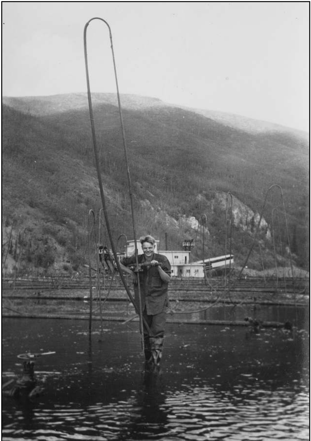
A dredge worker drives points in a thawing field while the Coal Creek dredge works the previous year's melted gravel. The steel piping of a thawing point was long because it needed to melt up to twenty-five feet down. (AH)
