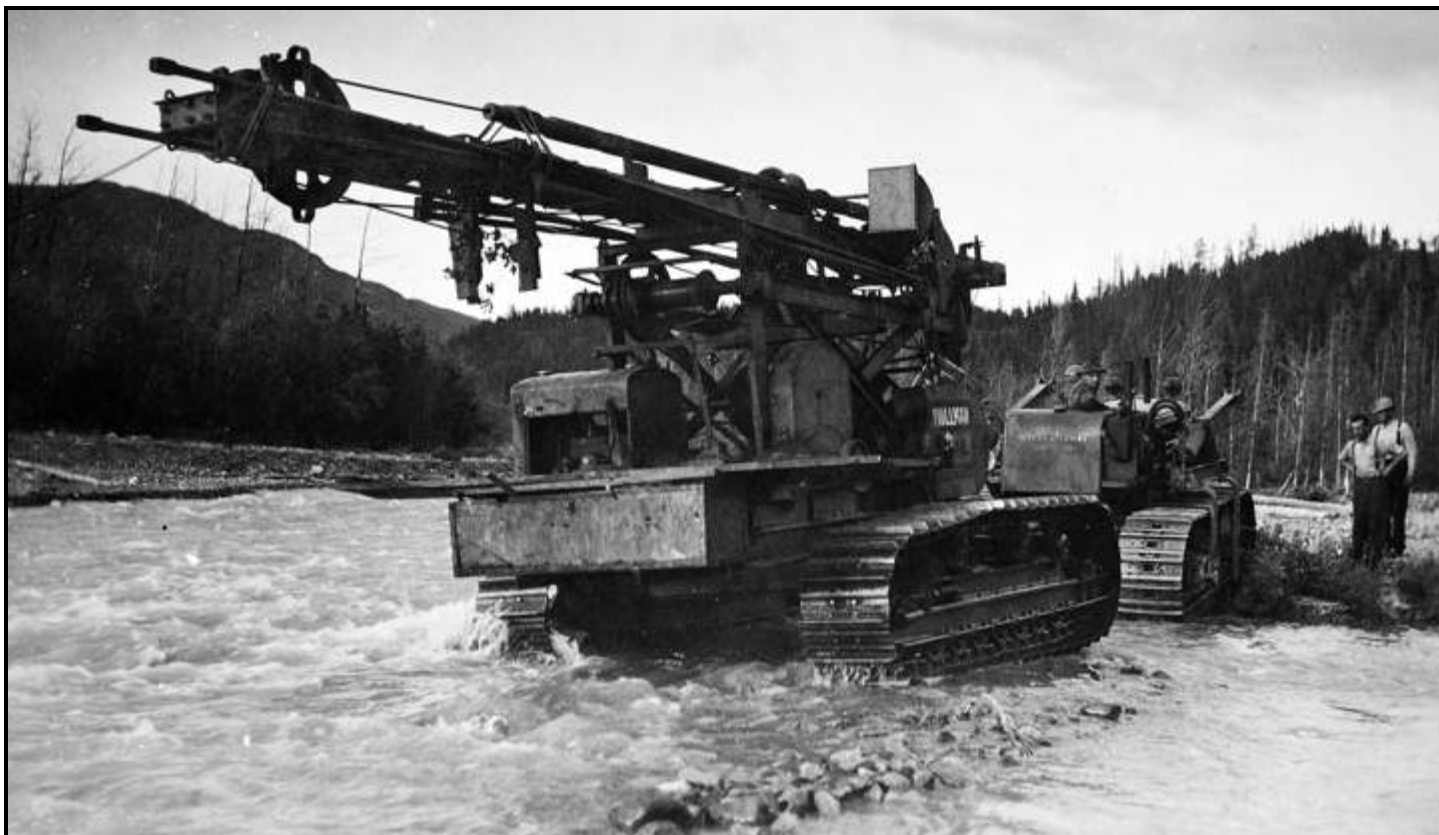
The "Prospector" by C. Kirk Hillman was a churn drill capable of moving with tracks over rugged terrain. This drill and the "Airplane" model were used to create maps of gold values at Coal Creek, Woodchopper Creek, and beyond. (SP)
