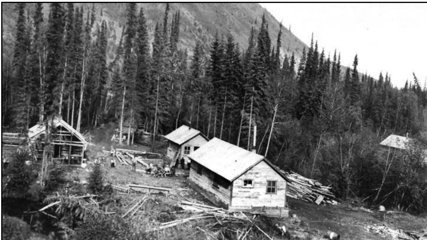
The earliest camp buildings at Coal Creek were a combination of log cabins and frame structures. The logs were local, but the materials for the rest of the buildings arrived from California via Yukon River steamboat. (EP)
