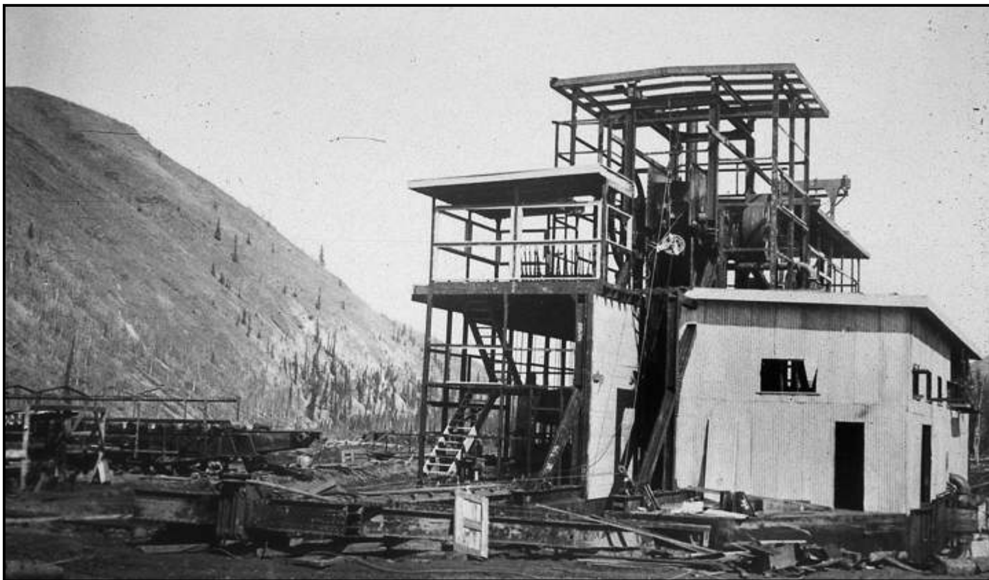
Ropes and pulleys were essential for lifting heavy dredge parts into place; the siding has been installed on the port side and soon the bucket line (parts seen at far left) will be lifted into place. (WL)
