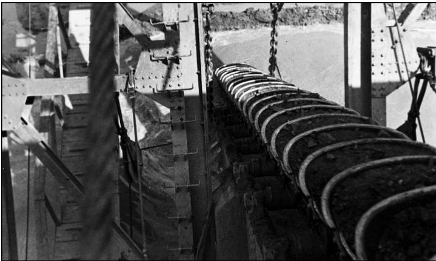
The dredge's sixty-two buckets could be raised or lowered to find the richest layer of gold-bearing gravels, and the work continued non-stop until late October or early November when sub-zero weather ended the season. (AH)
