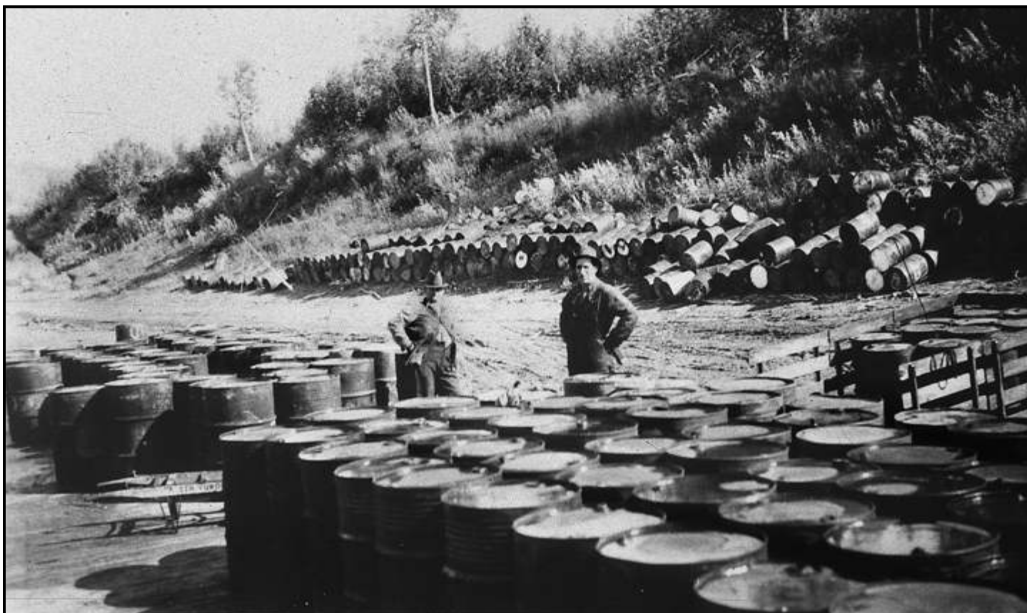
Jim McDonald and Bill Lemm watch over a stockpile of fuel barrels on the landing below Slaven's Roadhouse. The two Atlas generators on the Coal Creek dredge used 180 gallons of diesel each day, and more was needed to keep the tractors running. (WL)
