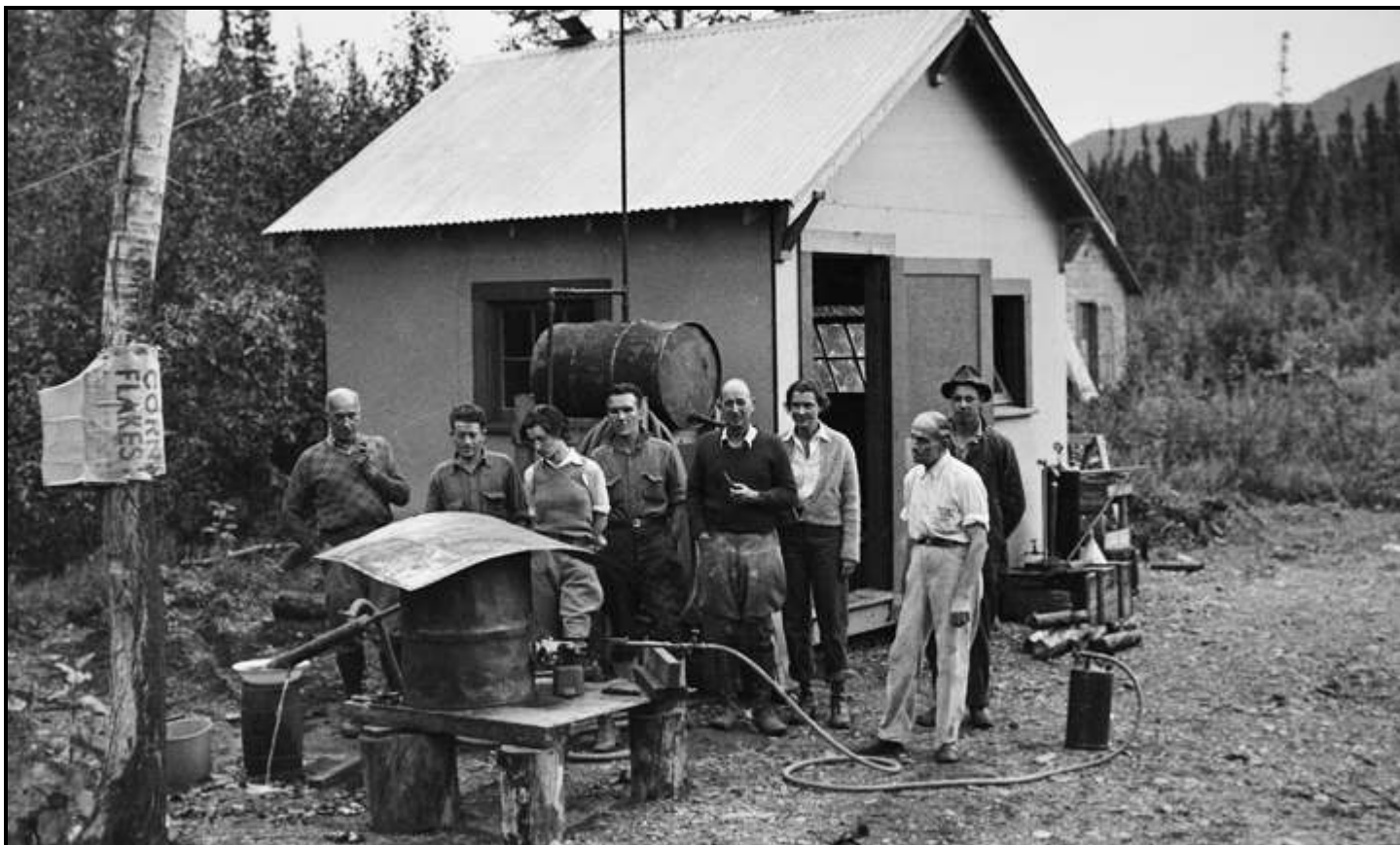
Alexander McRae (left), Ernest Patty, and others gather to observe the first step in refining gold from the dredges. In a retort, they heat a mixture of gold and mercury until the mercury vaporizes leaving behind a “sponge” of gold and other minerals. (SP)
