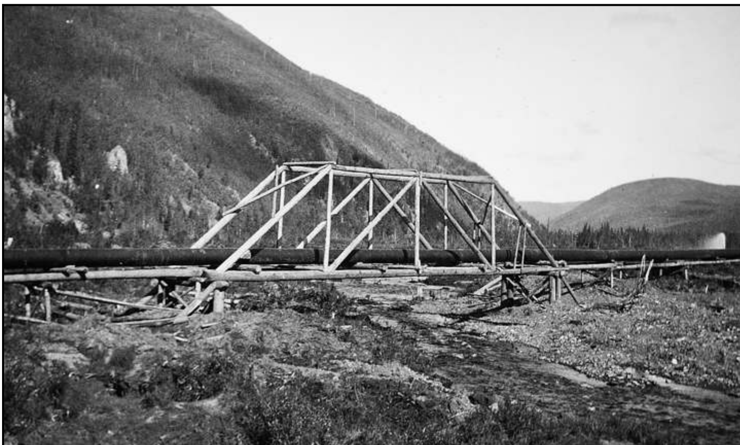
This temporary bridge supports a pipe carrying water under pressure across a portion of Coal Creek. As the dredge moved along the creek drainage, this bridge would be dismantled and erected elsewhere. (SP)
