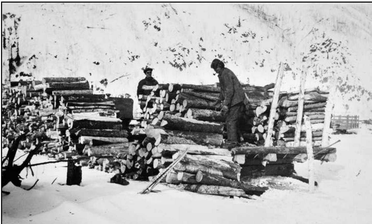
Dredge workers were never idle. Here they cut and stack cordwood to fuel the steam boilers mounted inside each dredge. The boilers helped to melt ice that built up inside the dredge in Spring or Fall when temperatures dropped. (SP)
