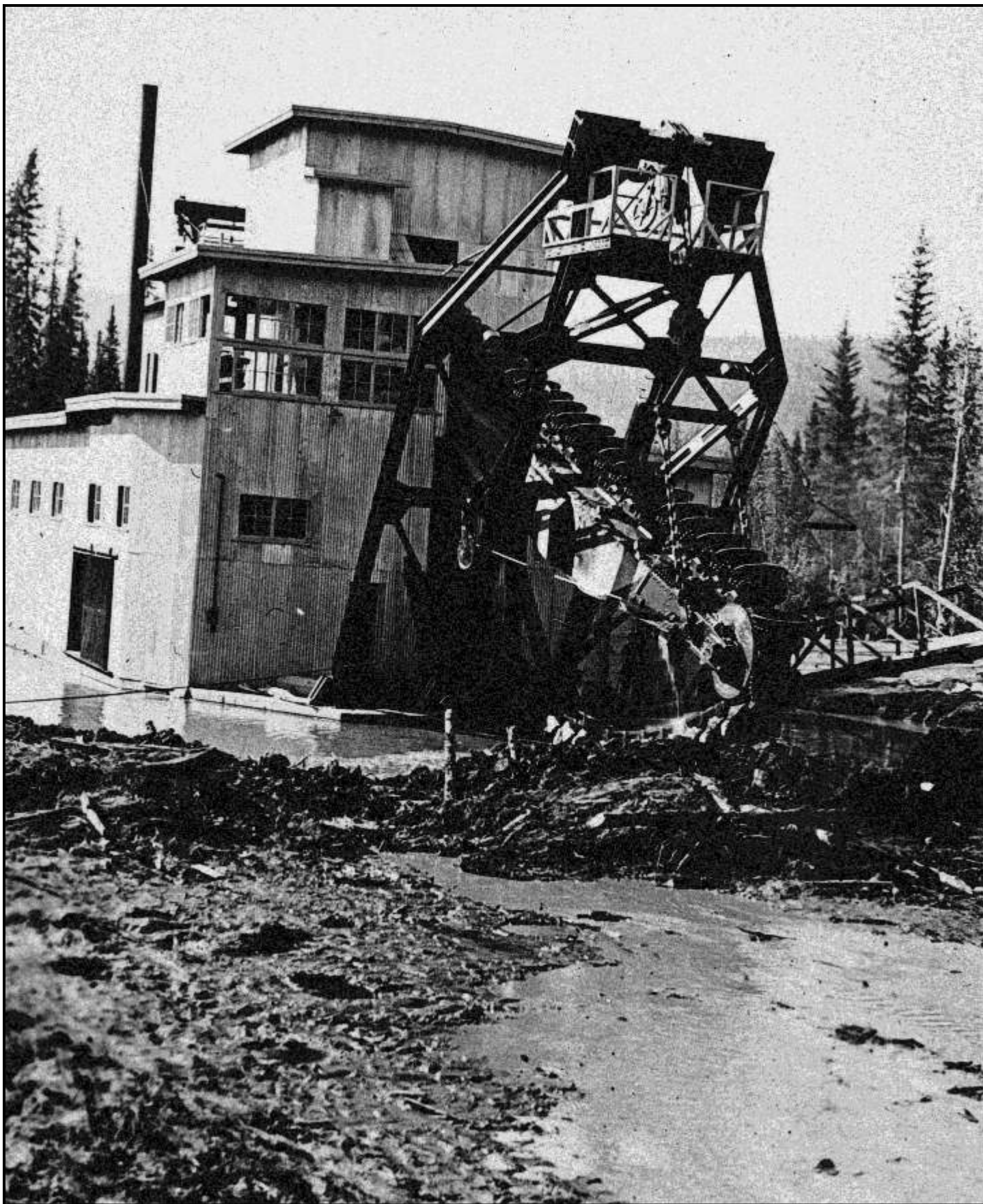
The Coal Creek gold dredge on its first full day of operation, July 1, 1936. General Manager Ernest Patty later wrote, "Its two diesel engines began coughing; the winchman moved the dredge out of the construction pit and the bucket line started to revolve and bite into the gravel. It was a great moment to hear the thump of the first gravel falling into the hopper." (EH)
