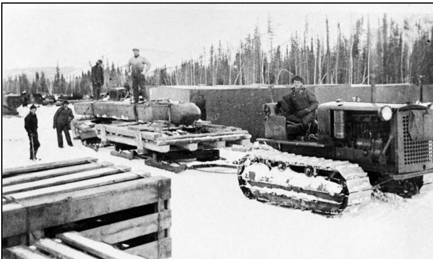
Workers transport the 40-foot-long "spud" weighing nearly seventeen tons to the dredge construction site. The spud, installed at the rear of the dredge, served as an anchor and pivot point that could be raised or lowered as the dredge advanced. (GB)
