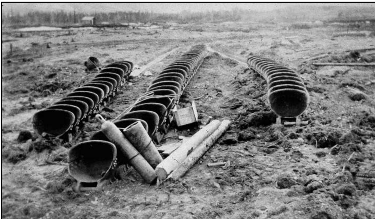
Dredge buckets, each capable of holding four cubic feet of material, wait to be installed. Each season, the digging edge of the buckets was worn away from constant use, so the buckets were designed with replaceable lips. (WL)
