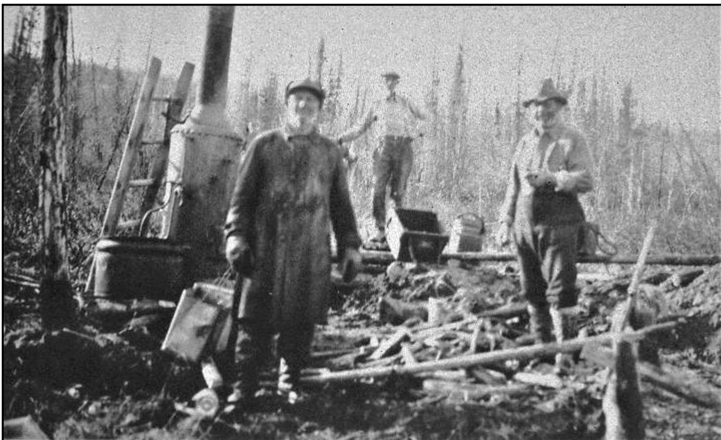
Frank Slaven (foreground) and other old-timers prospecting for gold near the Charley River. They are using a steam boiler to melt frozen ground and buckets to bring the gravel to the surface. The ladder next to the boiler emerges from their mine shaft. (WL)
