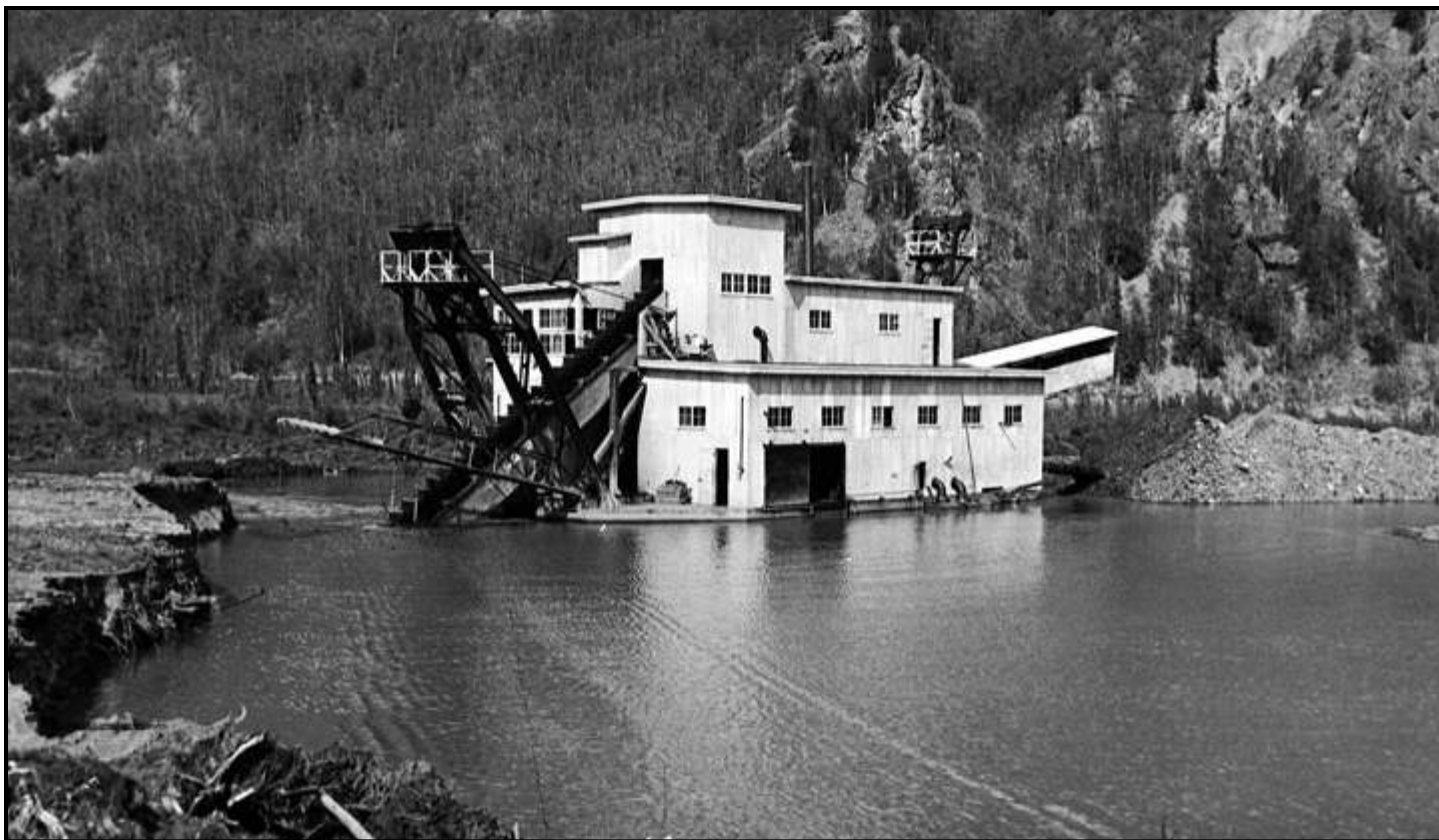
Once in operation, the dredge floated in a pond of its own making, and as it excavated gravel, long steel cables attached near the bow were used to pull the machine left, right, or forward. Note ripples in the water where a cable slipped beneath the surface. (SP)
