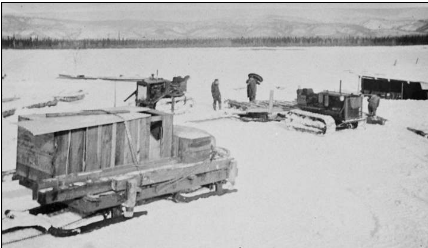
In early March 1936, tractors and sledges on the bank of the Yukon River prepared to move dredge parts up Coal Creek to begin construction. Moving heavy loads overland was easier over snow and when the ground was still frozen. (GB)
