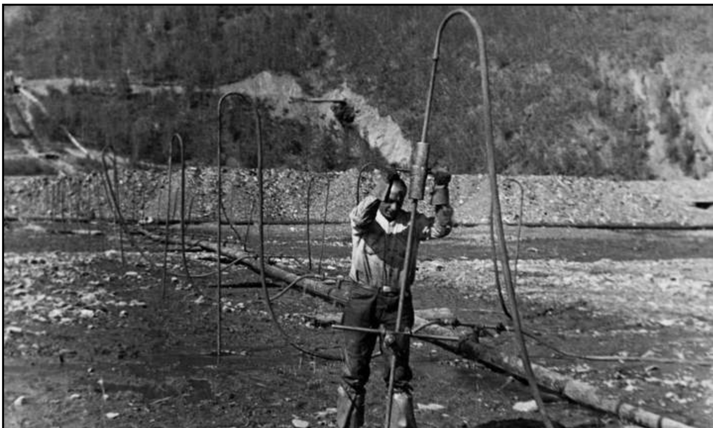
Thawing points were equipped with a “hammer and anvil” system, which allowed a worker to drive the chisel bit a few inches at a time into melting permafrost. The work was backbreaking and made more difficult by mosquitoes and standing water. (AH)
